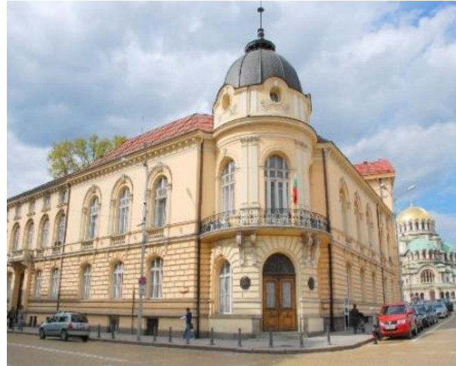
The building of BAS nowadays
